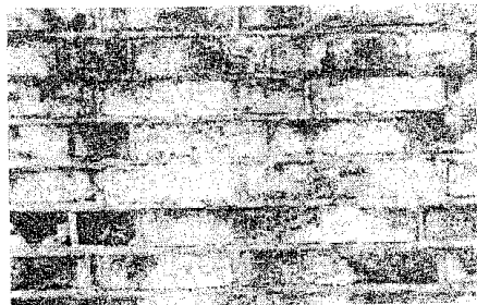
Figure 7-Checking and Cracking
